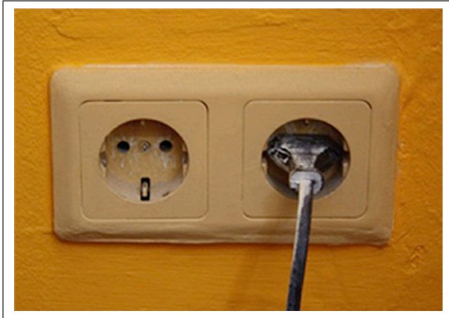
Figure 2. The Dutch 'Schuko' two-pin socket with a 'Europlug' inserted. © Photograph: Damon Taylor.
